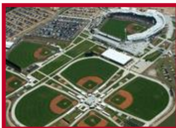
"Premium turf installed by 1776 Construction Group at JetBlue Park, the Spring Training home of the Boston Red Sox."
