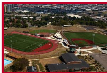
"Top-tier turf installation by 1776 Construction Group for Belmont University's Division I Baseball and Soccer programs."
